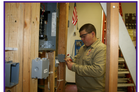
Electrical Maintenance Student working on wiring techniques.
