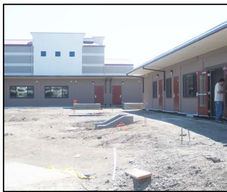
MC Village under construction.
